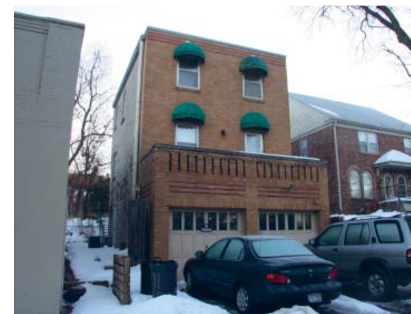
Apartment building at 811 South 60th Street (DO09:0428-010)
