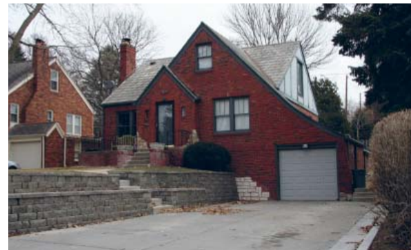
Minimal Traditional house with Tudor Revival influences located at 1507 South 58th Street (DO09:0424-013)
