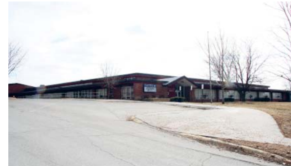
Belle Ryan Elementary School at 5845 Walnut Street, DO09:0424-025
