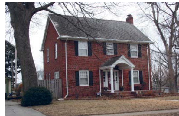
Colonial Revival house located at 1025 South 52nd Street (DO09:0427-031)
