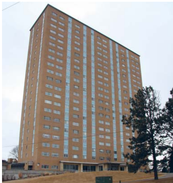
Elmwood Tower at 801 South 52nd Street (DO09:0427-025)
