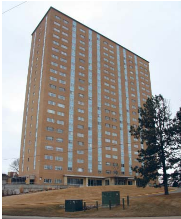
Elmwood Tower apartment building at 801 South 52nd Street, DO09:0427-025
