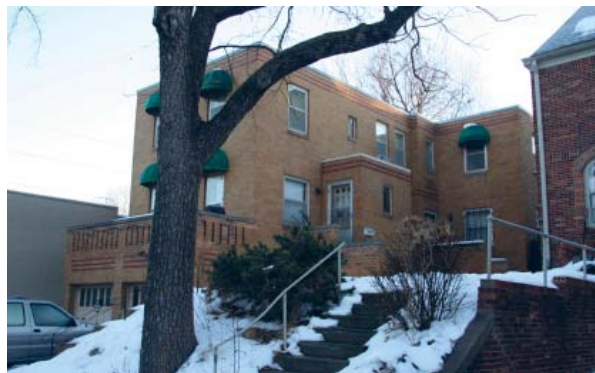
Apartment Building at 811 South 60th Street, DO09:0428-010
