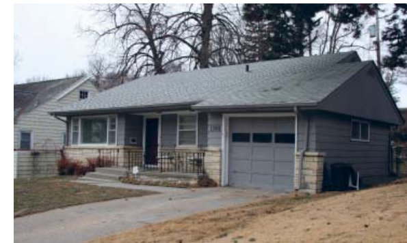
Ranch-style residence at 1508 South 58th Street (DO09:0424-014)
