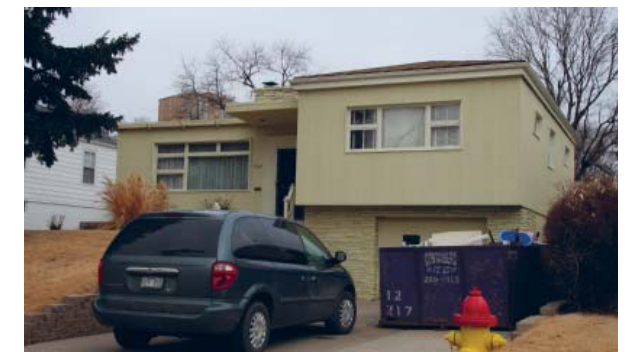
Contemporary residence at 5024 Pierce Street (DO09:0425-015)
