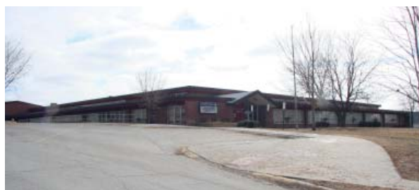
Belle Ryan Elementary School located at 5845 Walnut Street (DO09:0424-025)
