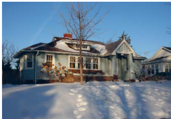
Craftsman house located at 854 South 59th Street (DO09:0428-016)
