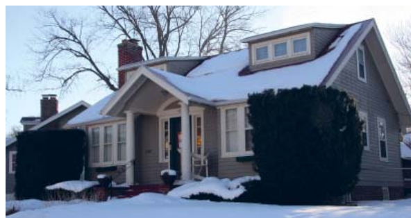
5805 Rees Street in the Edgewood Addition (DO09:0428-017)
