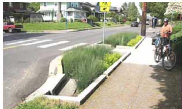
Bioswale Curb Extension Portland, Oregon
